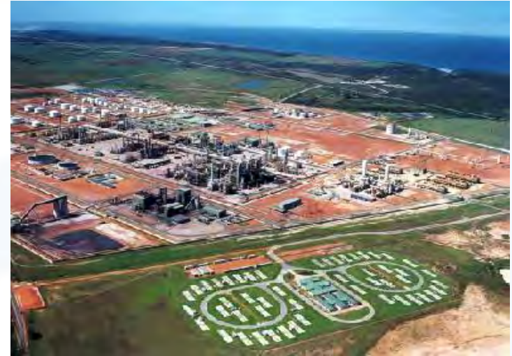
PetroSA GTL Plant, Mossel Bay, South Africa – courtesy of PetroSA
